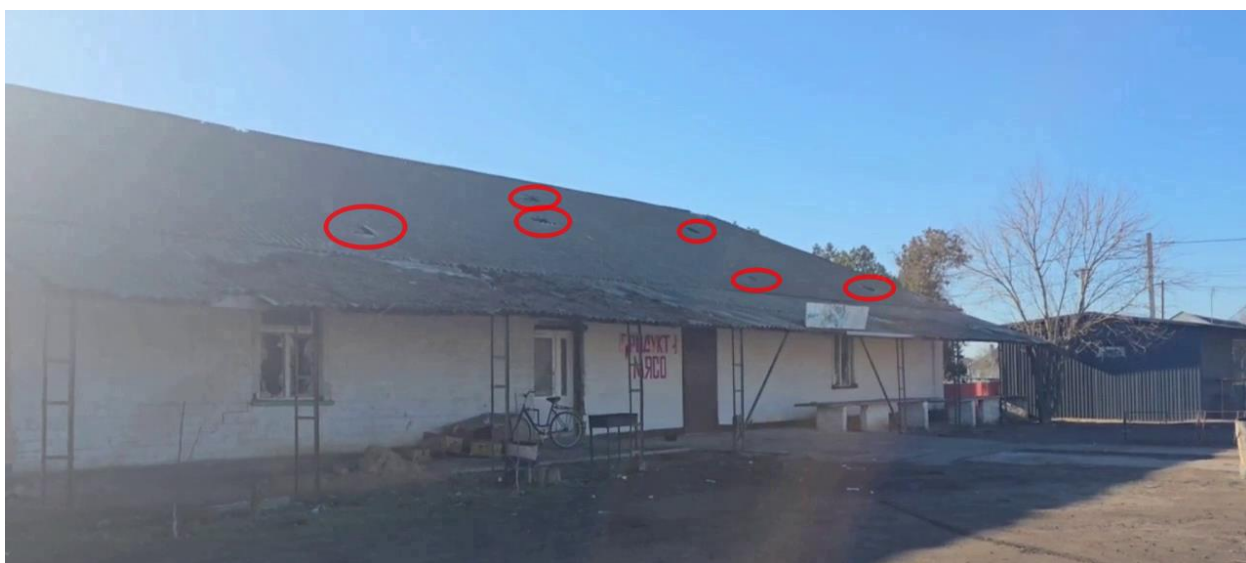
Fig. 8 - Holes from the CSM detonation on the roof of a one-story building north of the school building in the village of Bekhtery.
