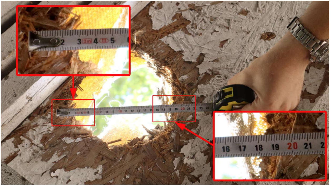
Fig. 20 -Measurements of the diameter of the hole in the roof at the site of shell hit 11.
