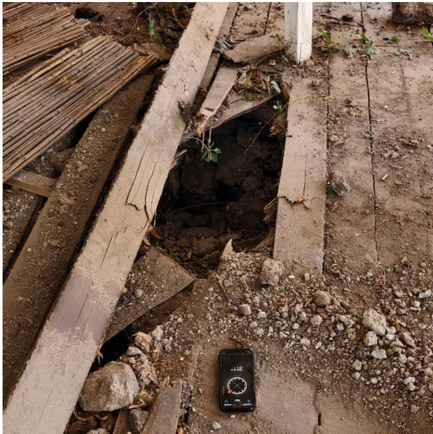
Fig. 28 - Shelling direction determination at the site of shell hit 11.
