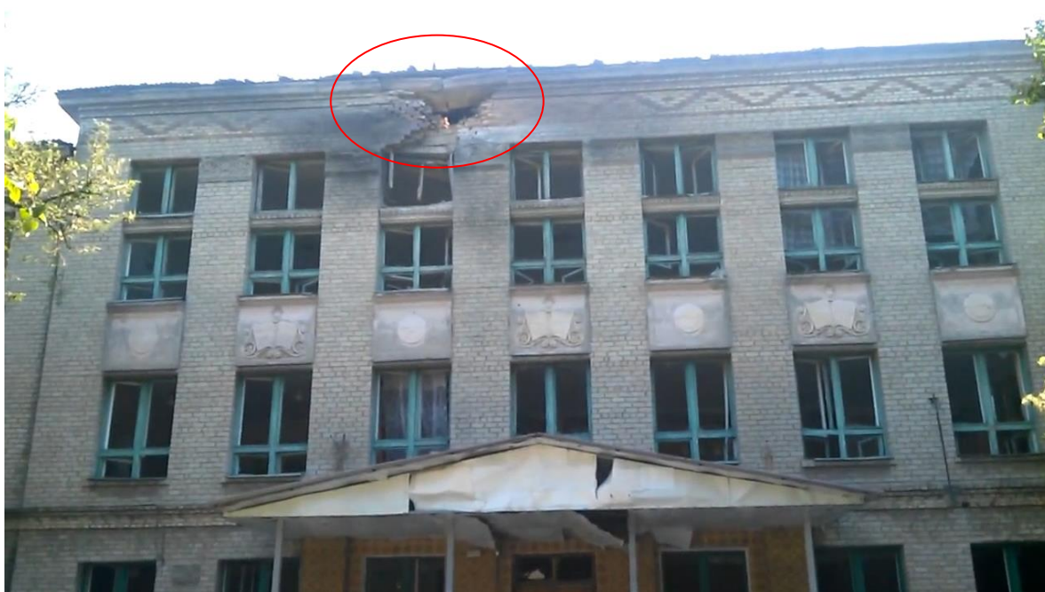
Figure 8. General Secondary School No 85, Horlivka 27.07.2014. 8
