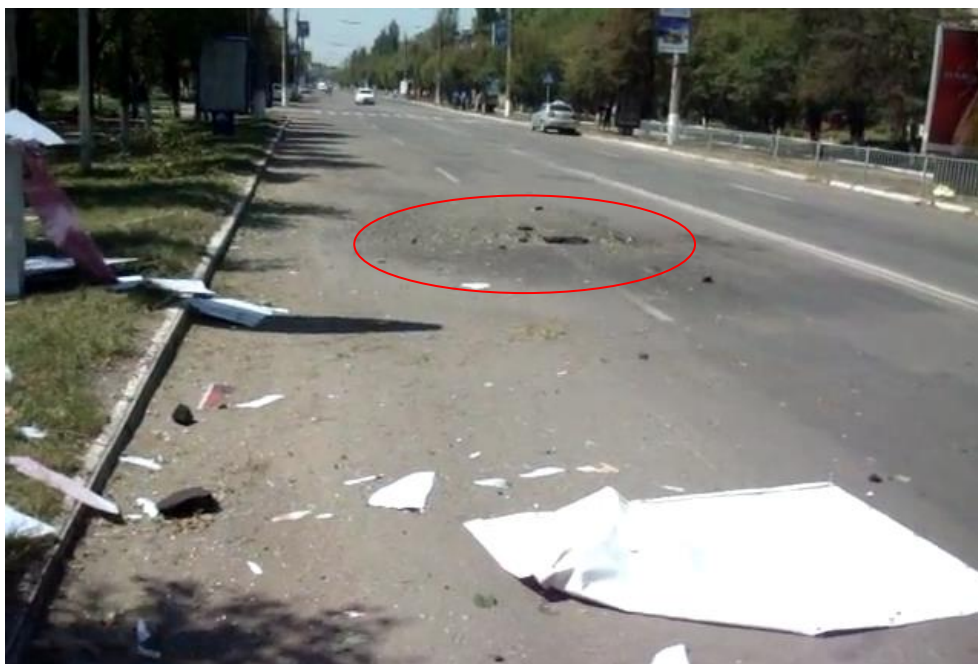
Figure 5. A crater from shell hit on the asphalt pavement opposite the residential building at 48, Pobedy Ave., Horlivka, 27.07.2014. 5
