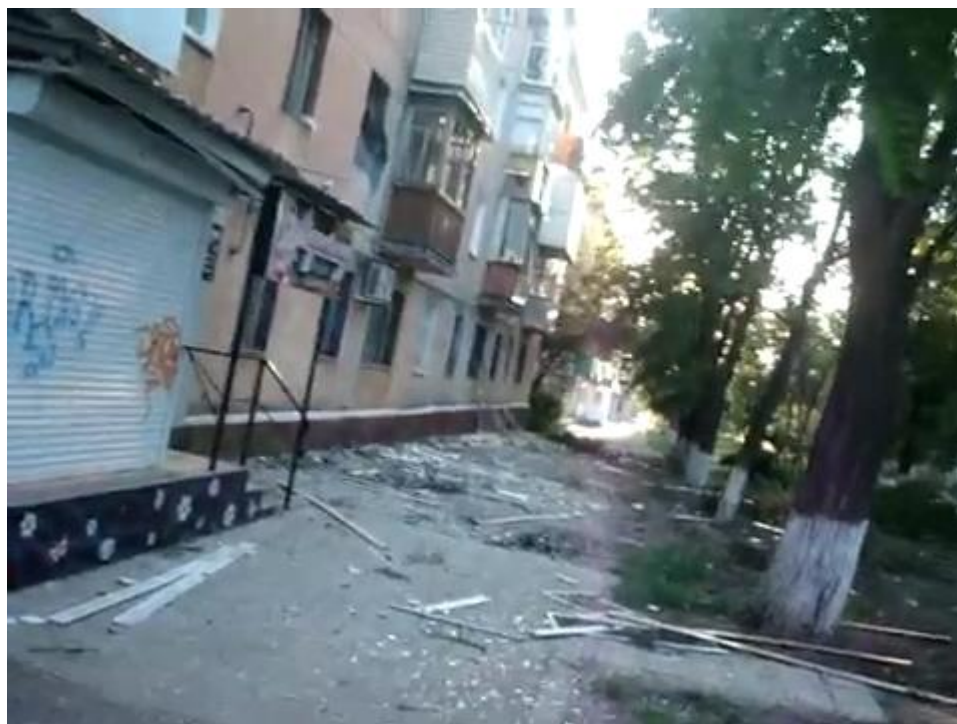
Figure 7. Residential building at 50, Rudakova St., Horlivka, 27.07.2014. 7
