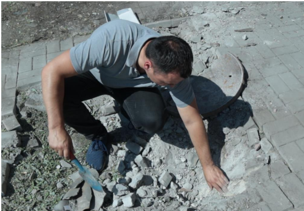
Fig. 5 – Inspection of the crater from a shell explosion near building No. 43 in Chelyuskintsev Street.
