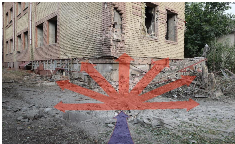
Fig. 12 – Direction of the main scatter of fragments in the case of shell hit 2.
