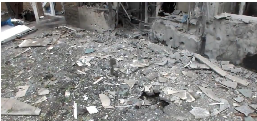
Fig. 7 - Shell hit (No.4) near the entrance to the “Chubchik” hairdressing salon at 10, Gvardeisky quarter 9 .
