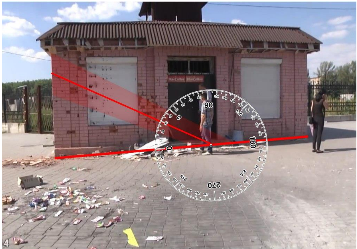
Fig. 28 - The trace from the main scatter of fragments on the wall of the Kosheliok food store.
