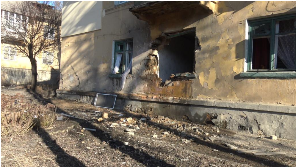
Fig. 4 - The traces of the projectile hitting in the residential building at 3, Semionova-Tyan-Shanskogo St.
