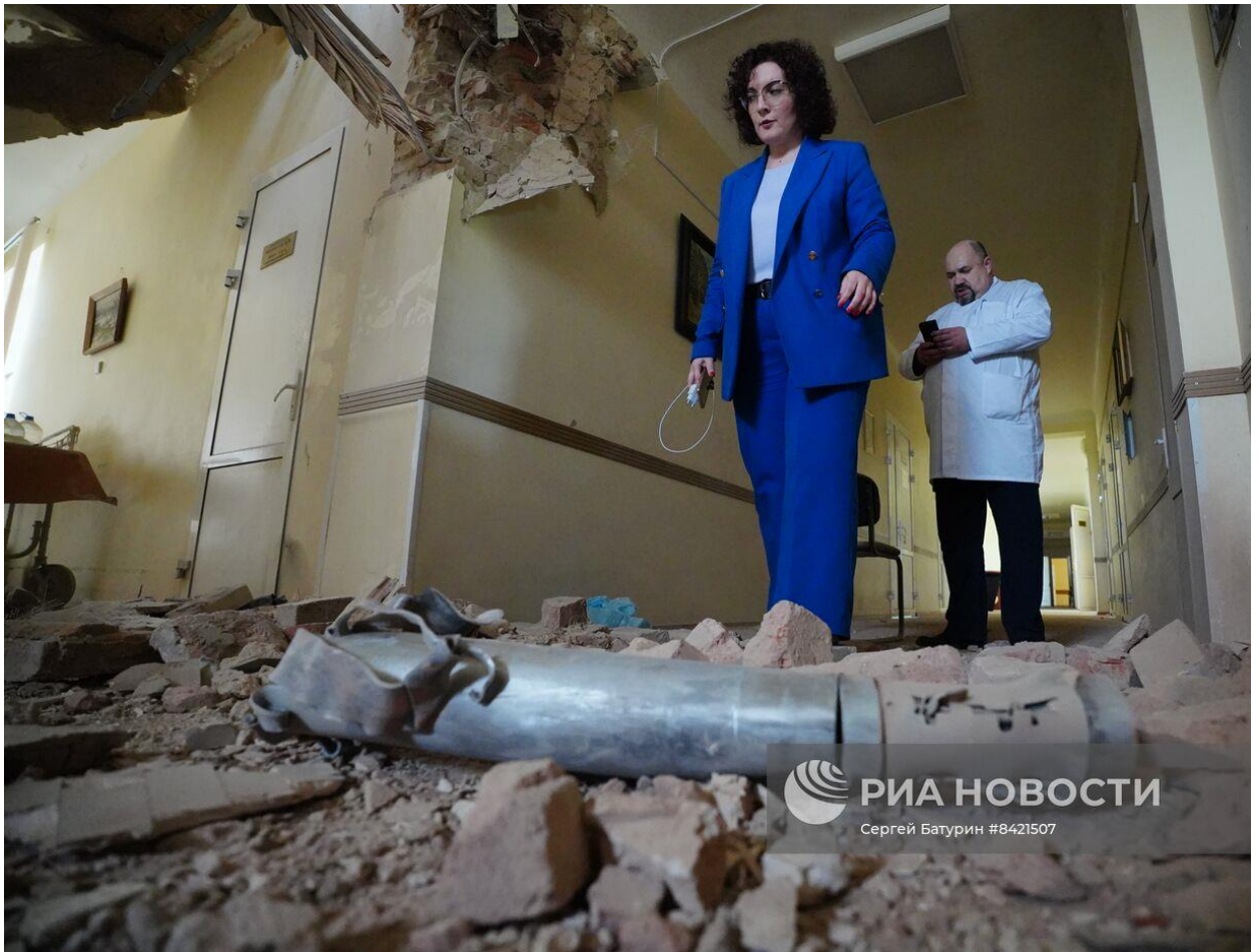
Fig. 35 – The rocket projectile that damaged the main building of the Republican Traumatological Center 36 .
