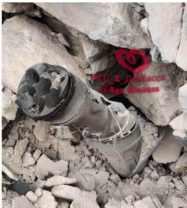
Fig. 30 – Debris of a rocket projectile in the basement of the multi-apartment residential building at 10, Donbass Liberation Ave 32 .
