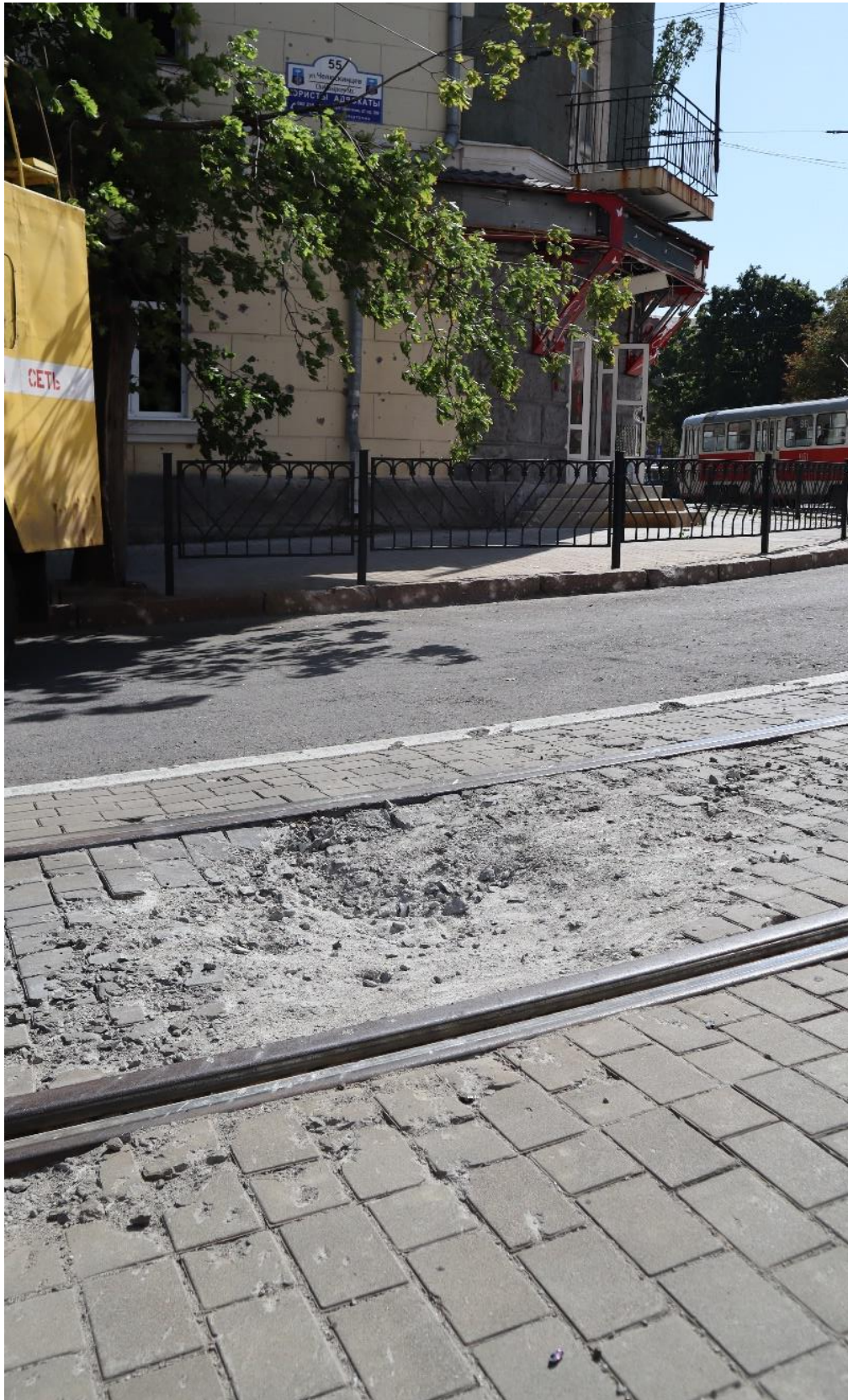
Fig. 11 – An artillery shell explosion crater between the tram rails next to the residential building at 55, Chelyuskintsev Str.
