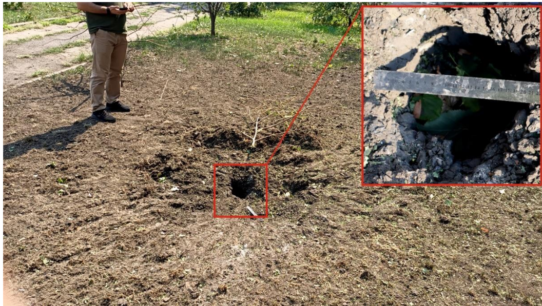
Fig. 5 – An artillery shell explosion crater next to the residential building at 3, Constitution Square.
