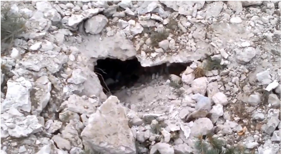
Fig. 25 – A crater from the shell in the car parking to the west of the building at 3GTimiryazev St., Luhansk 36 .
