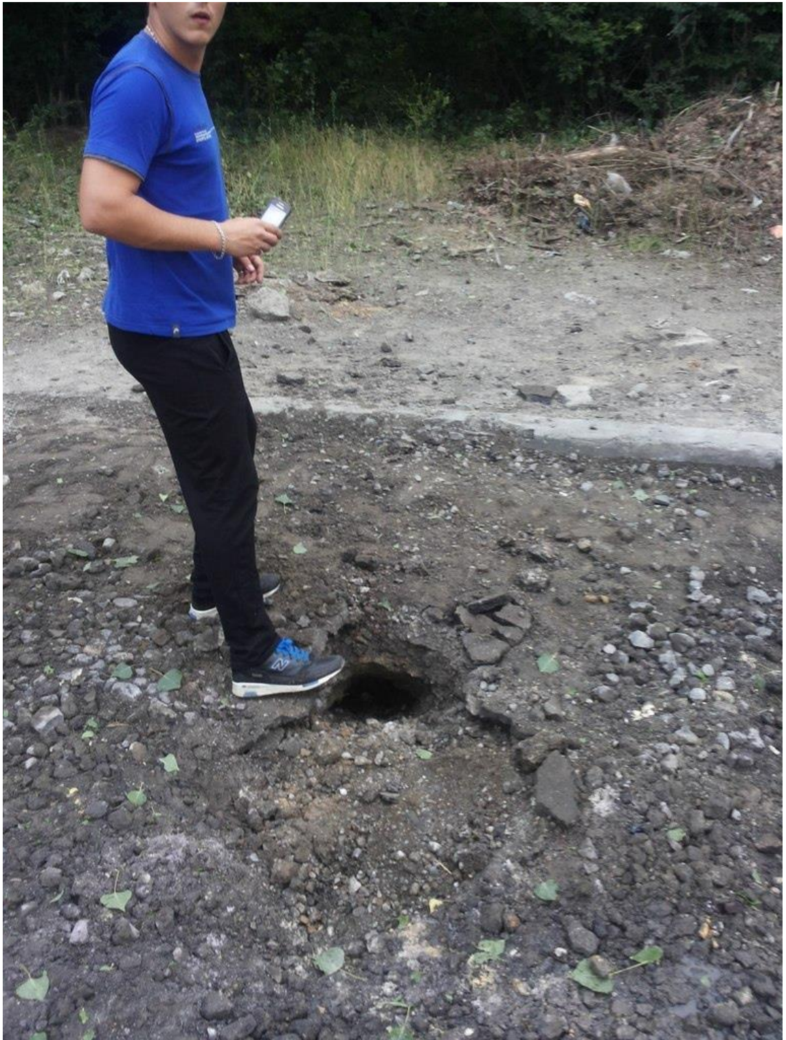
Fig. 29 - A shell explosion crater located about 25 meters from the south-western corner of the building at 3G, Timiryazev St., Luhansk 39 .
