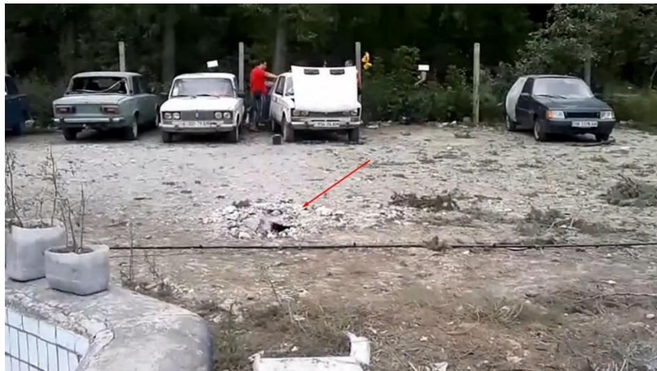
Fig. 24 - A crater from the shell in the car parking to the west of the building at 3G Timiryazev St., Luhansk 35 .
