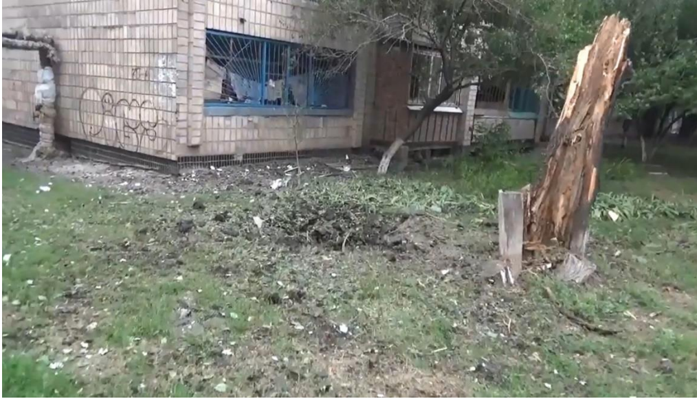
Fig. 13 - An artillery shell explosion crater on a lawn a few meters from the south-western corner of a multi-storey residential building at 79A, Andrey Linyov St, Luhansk 25 .
