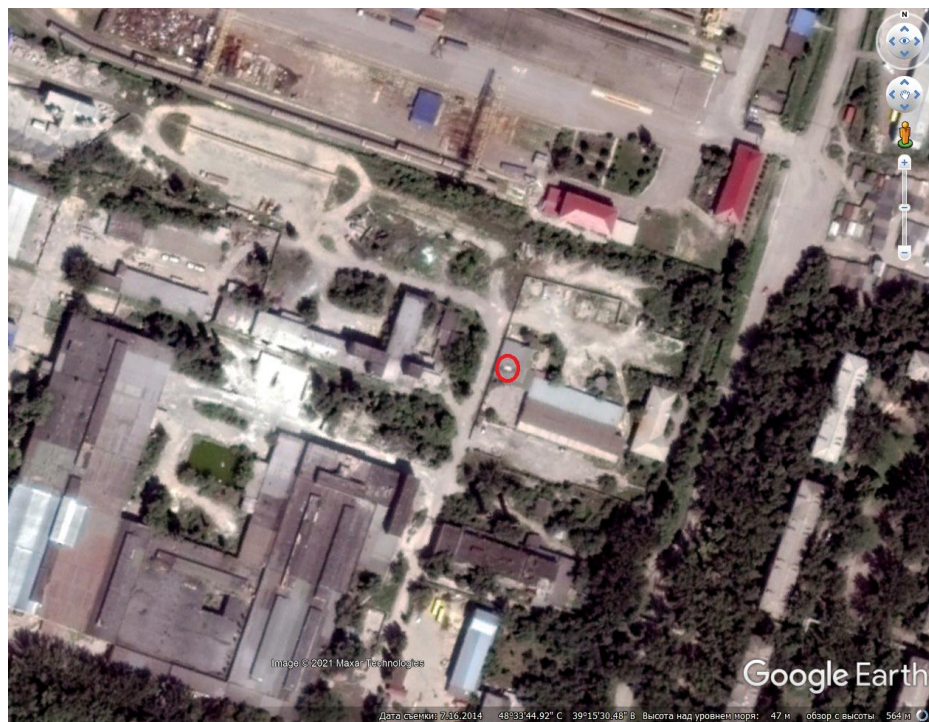
Fig. 28 – Trail of the shell hit into the roof of the utility premises located to the north of the building at the address 75 lit Z, Andrey Linyov St., Luhansk, satellite image dated 16.07.2014.
