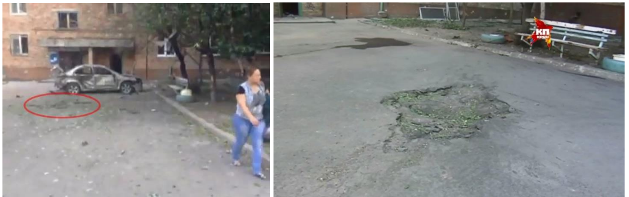
Fig. 3 – Shell hit No. 7: 23, Kutuzov Street. Left - general view against the background of the vehicle damaged by the blast 21 , on the right - the crater itself. 22
