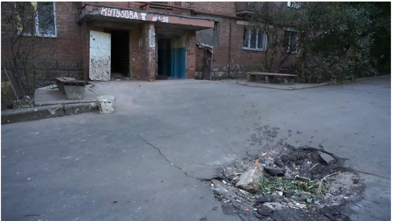
Fig. 14 – Shell hit No. 14: 7, Kutuzov St. 32
