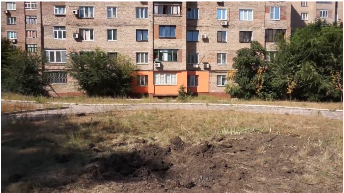
Fig. 5 - Shell hit No. 9: approximately 25 meters south of building No. 25 in Kutuzov St. 24
