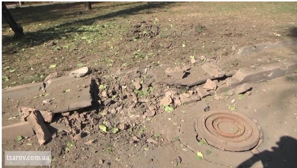
Fig. 16 – The site of the shell hit in the pedestrian footpath about 20 meters north of the northern part of a multi-storey residential building at 77, Shevchenko Blvd. 43 .
