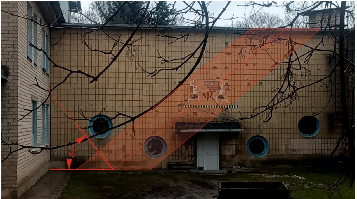
Fig. 24 – Determination of the angle of a projectile arrival based on the trace of the main scatter of fragments on the wall of the building of educational complex No. 16.
