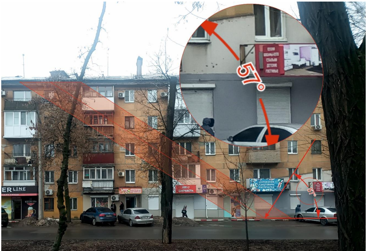
Fig. 23 – Determination of the fragment scattering angle (shell hit 7).
