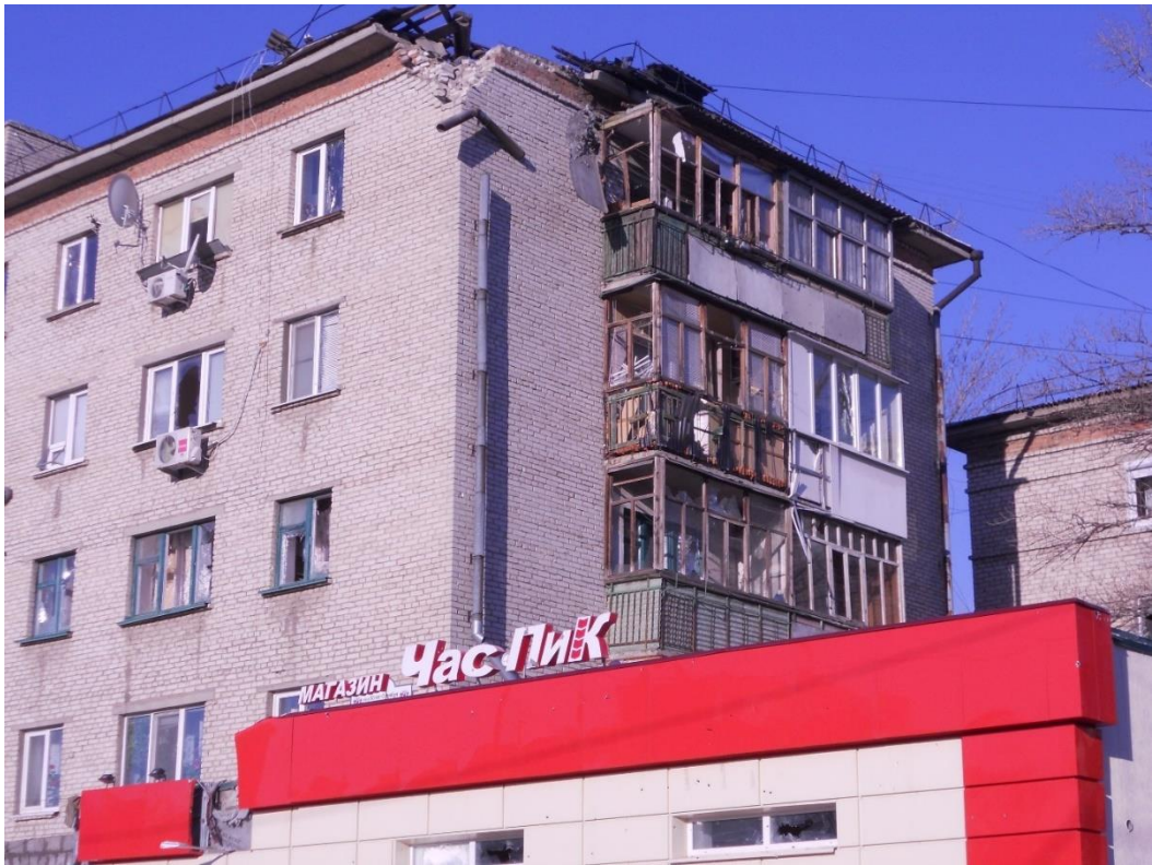
Fig. 8 –The eastern corner of the residential building destroyed as a result of shell hit 5 37 .
