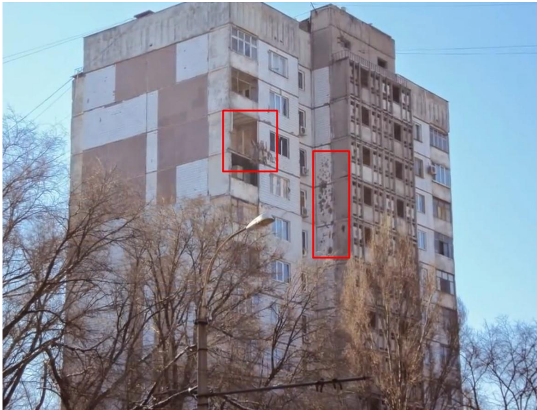
Fig. 11 – Destroyed balcony and traces from the main scatter of fragments at the impact site of shell hit 7 40 .
