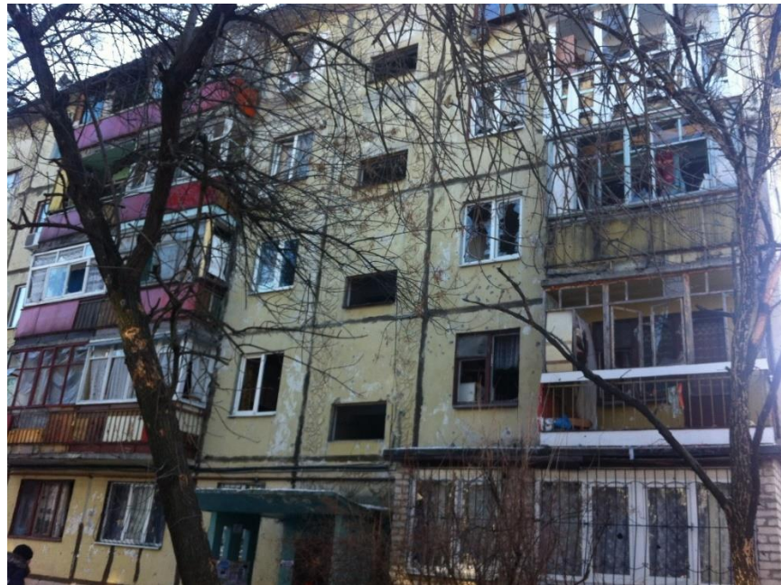
Fig. 15 – Consequences of a projectile detonation a few meters from shell hit 10 44 .
