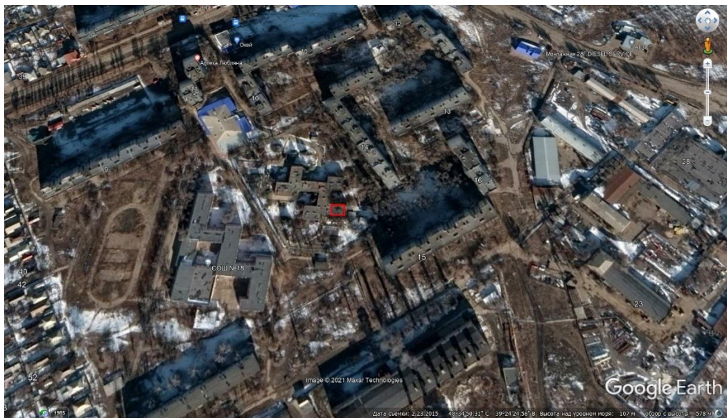
Fig. 3 – The trail of a shell hit 1 on the roof of Nursery School No. 129 on the satellite image dated 23.02.2015
